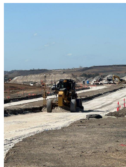
Photo of the internal road network, taken August 2023
