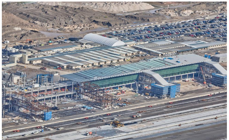
Aerial photo of the western pier and fixed-link bridges, taken August 2023
