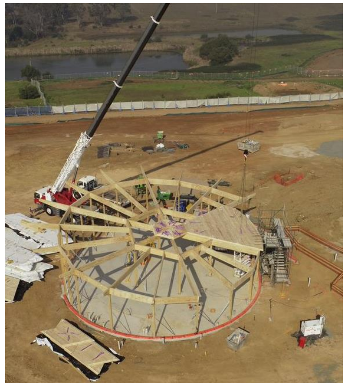
Roof installation, June 2019
