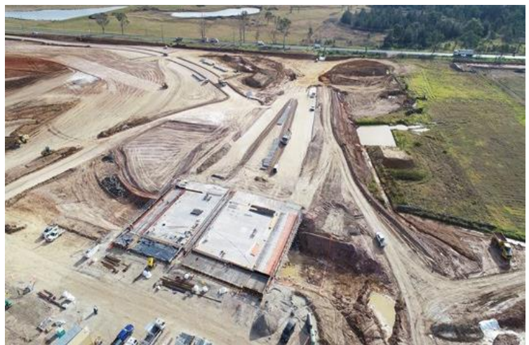
Badgerys Creek Road Realignment at Elizabeth Drive, July 2019
