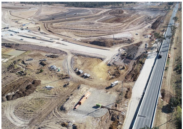
Badgerys Creek Road Realignment at Elizabeth Drive, August 2019
