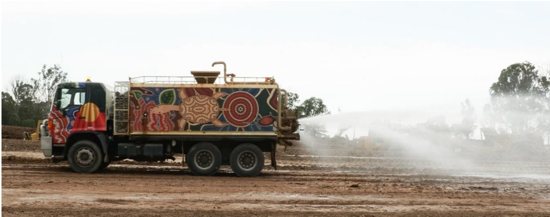
Watercart wetting earthworks site for dust suppression.
